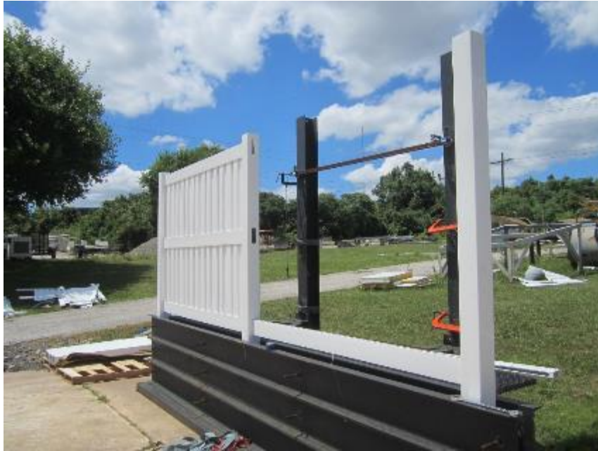
Photo No. 5 Specimen No. 2 Failure
